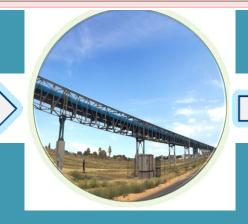
Cheapest, fastest conveying system 14.2 km length 4500 T/hr conveying capacity 5.6 m/s belt speed, Electric drive – VFD driven Environment friendly
